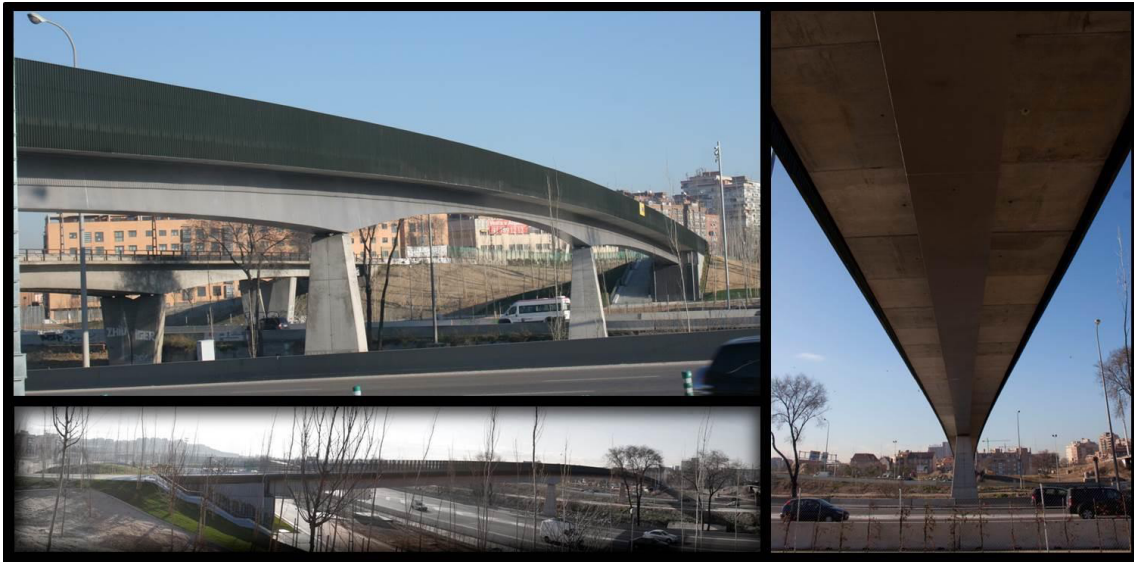
composite beam with variable depth, three 50m spans
